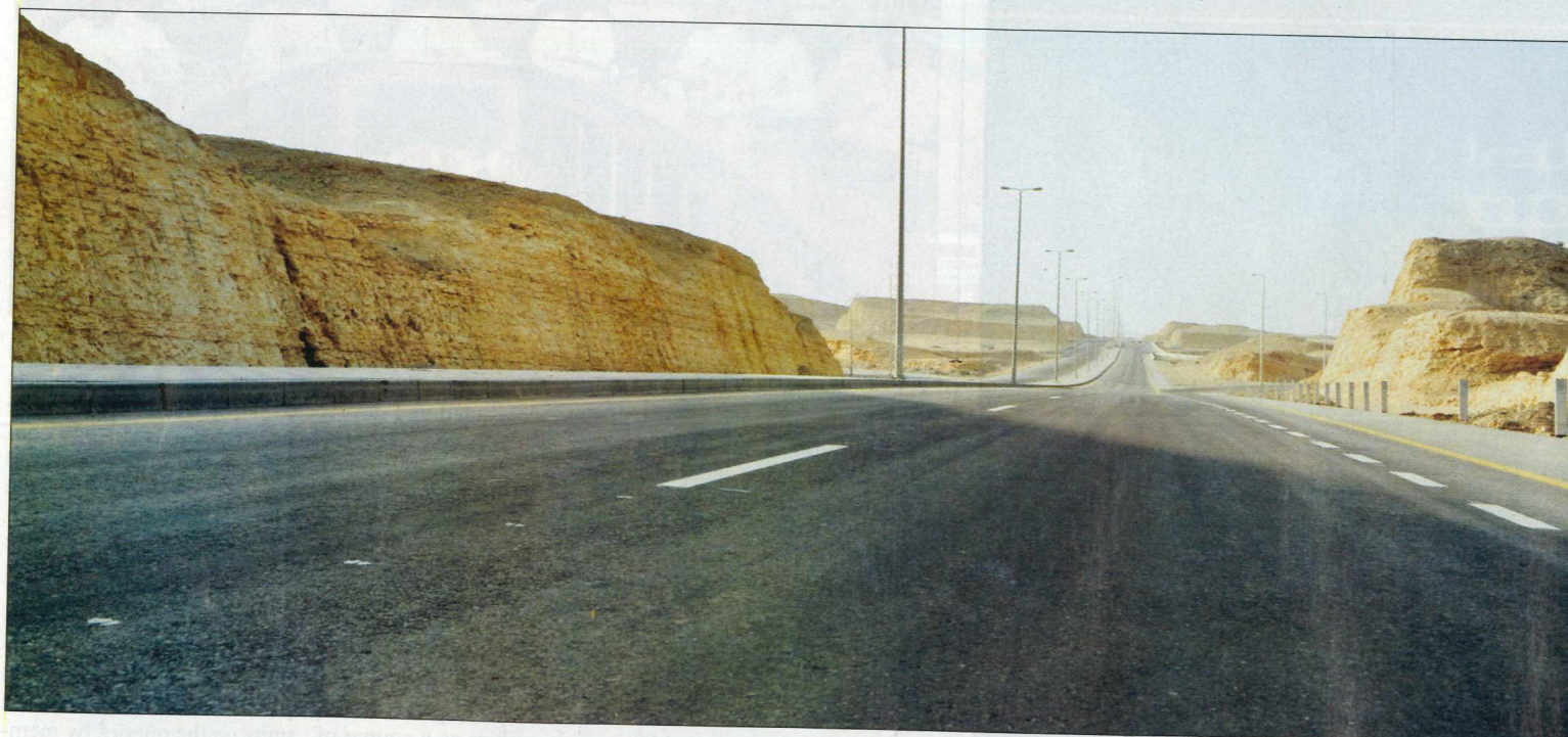
ROAD TO DEVELOPMENT: Forty-six days left for the opening of the Muscat Expressway, which is considered as one of the giant projects that would be opened to coincide with the Sultanate's 40th National Day. The Muscat Municipality lent great attention and exerted relentless efforts to design the Expressway, which contains high bridges matching the standard of world bridges. — Picture by Faisal al Balushi
